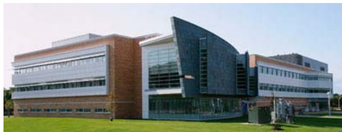
CEWIT's new building was opened in March, 2009 offers over 100,000 square feet of lab space.
